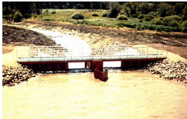
Figure 2. Weir after construction in 1986
